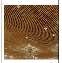
1.0mm, the supporting structure is to suspended using full threaded rod with minimum standards and Self-certified for its quality conformity. The Bamboowood products are to adhere to ASTM E 84 Class A standard and shall have a toxicity of less than 5 as per NES 713 standard. The Bamboowood planks shall have minimum density of 1000 kg/cum & minimum Hardness 1000 Kgf.
