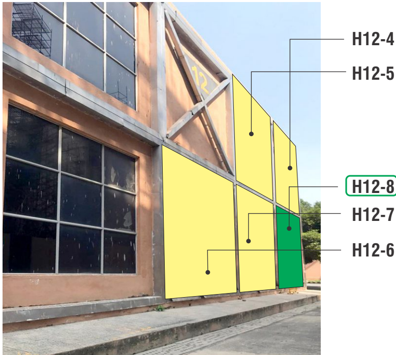
Location: Outer wall of Hall 12A, facing Halls 2-5
