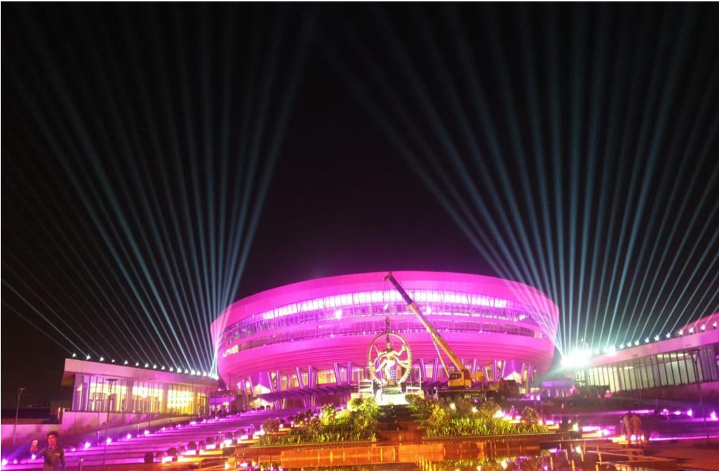
Sample Image of Façade Lighting at Bharat Mandapam (Indicative Image)
